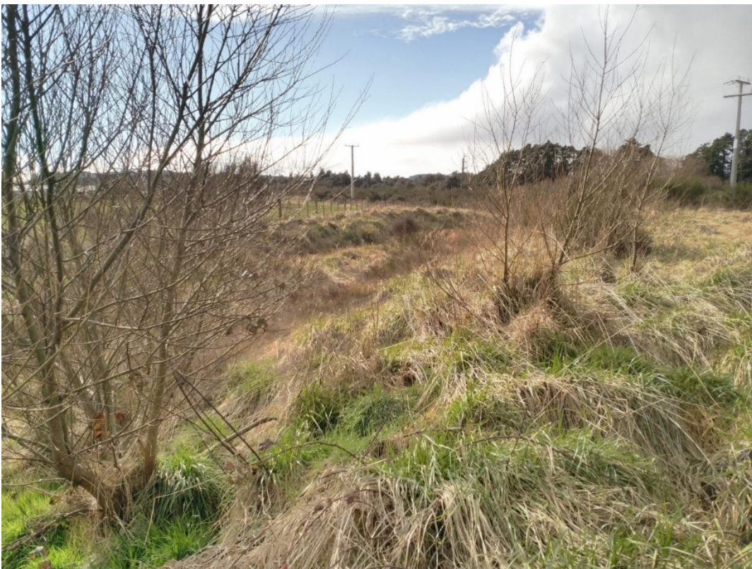
Photo 2: View of the Rangataua WWTP wetland looking upstream from the inlet point
