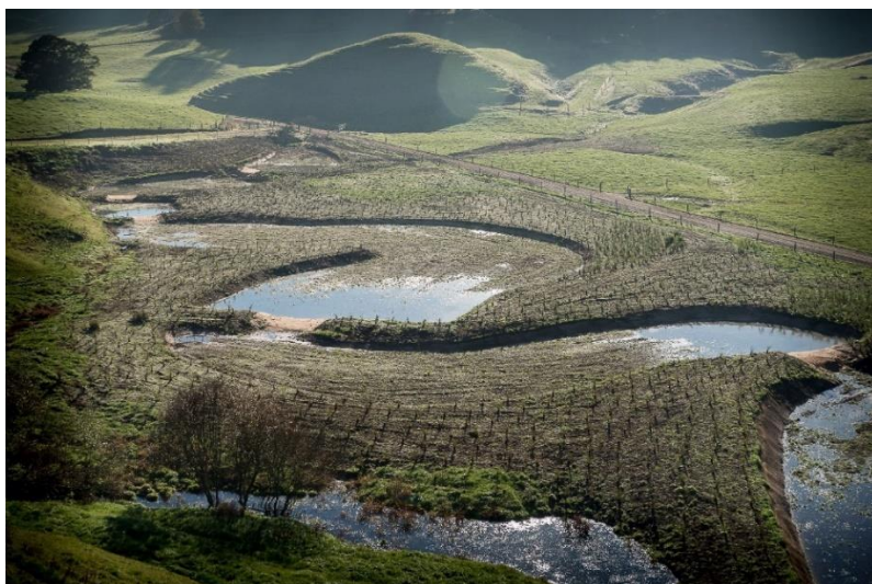
Figure 6: Constructed wetland showing wetland bays with coconut fibre reinforced sills set 500mm above the base of the upstream bay.
