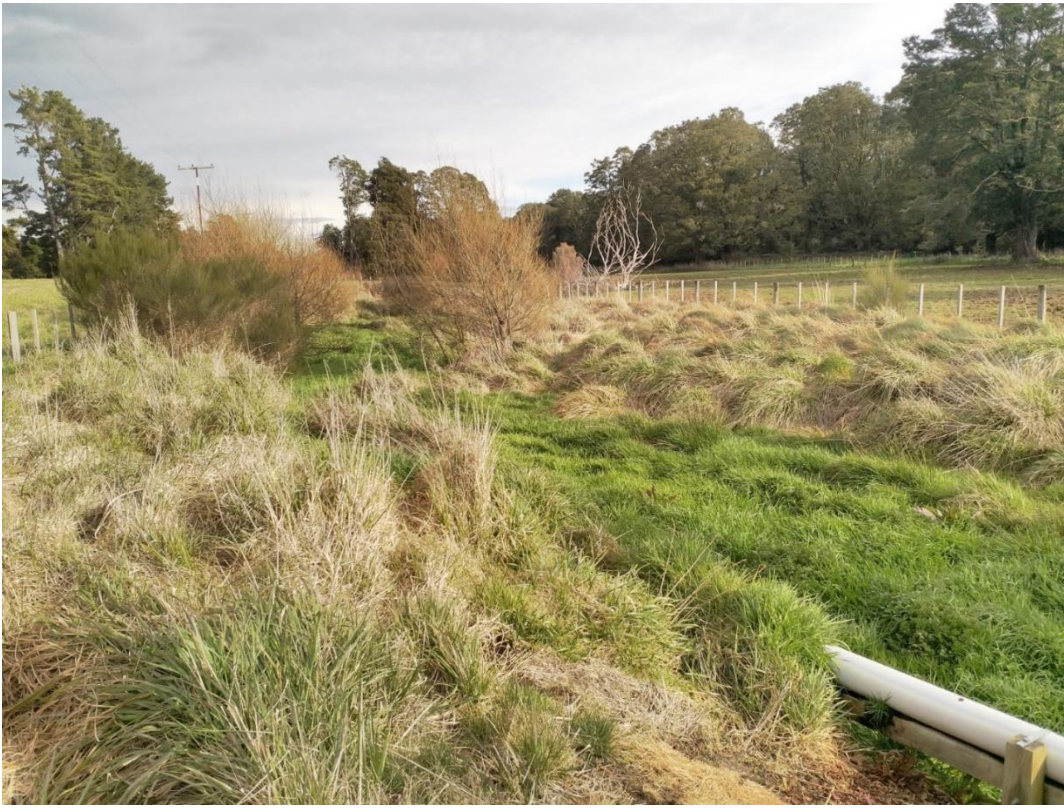
Photo 1 (above): View of the Rangataua WWTP wetland looking downstream from the inlet point
